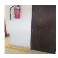
It was noted that 2 out of 05 fire extinguishers at production floor were mounted at improper height because it was about 2 meter from the ground to the fire extinguishers handle bar.
